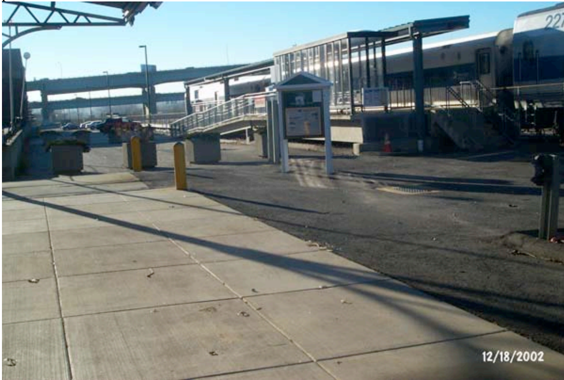
The Waterbury, CT, MTA Metro-North Railroad Station. I-84 is visible in the background.
