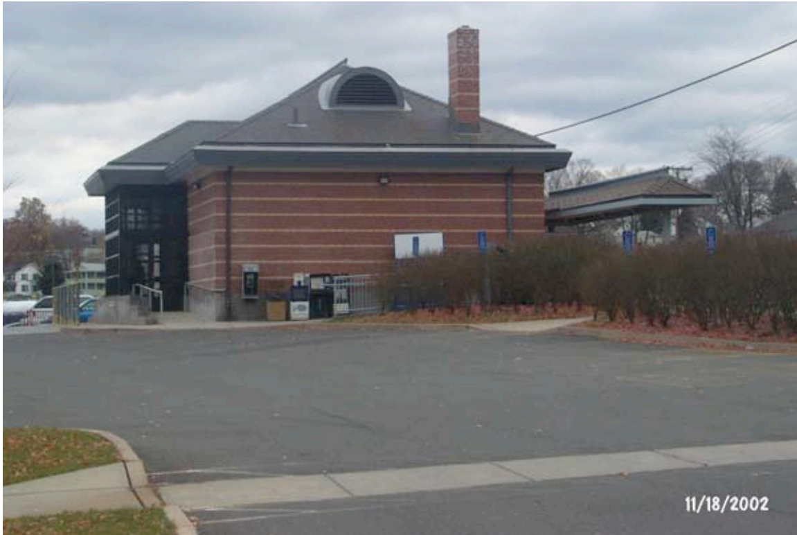
MTA Metro-North Railroad Station on Patriot Drive, Danbury
