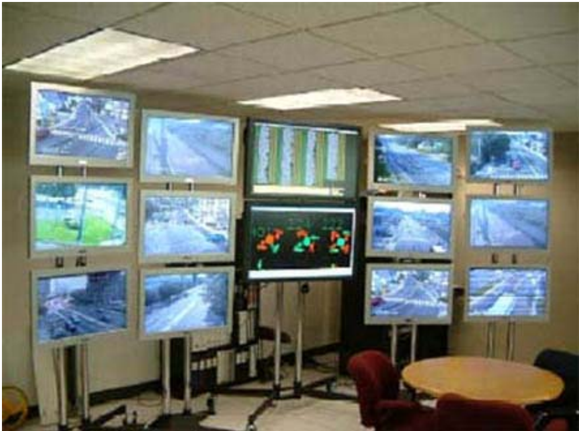
Figure 6.1 Stamford Central Traffic Control Room
