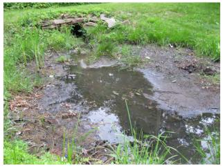
A basin where sediment has accumulated in the forebay and has killed off vegetation. Simple maintenance would improve the function of this structure and allow plants to use and filter the captured water.
