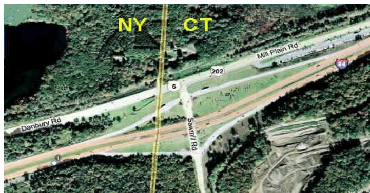
Yellow line is NY/CT border. I-84 eastbound traffic could too easily divert to Route 6 as the Exit 1 eastbound off ramp originates in New York State.
