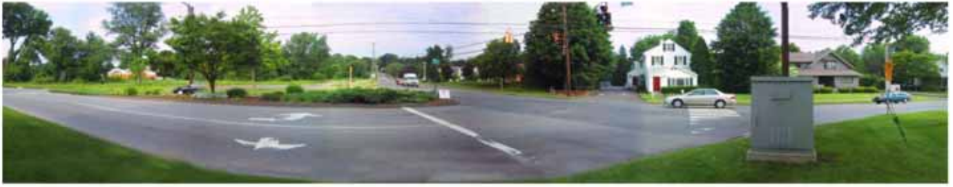
Existing: Intersection of Route 6 and Queen Street. (Queen Street northbound approach to Route 6)
