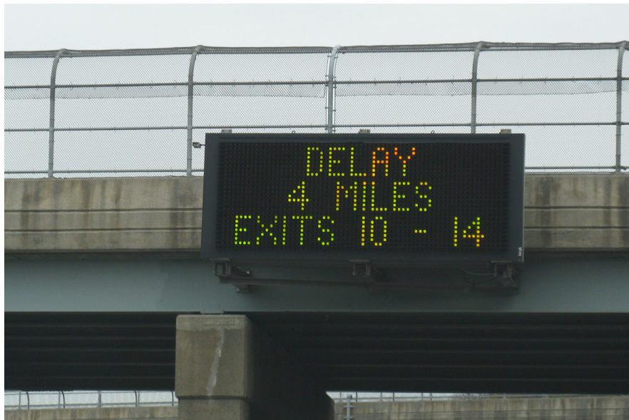
Photo 44: Changeable message signs, as seen on I-95, alert drivers about traffic conditions.
