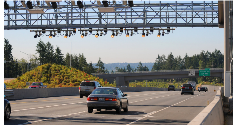
Photo 47: Any congestion pricing system deployed in the Region must use open road tolling technology, as shown below in this example from Washington State. Source: Washington Department of Transportation
