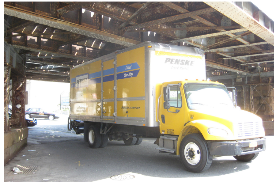
Photo 39: A disabled truck stuck under the Atlantic Street rail bridge in Stamford, one of many bridges with low clearances in the Region.
