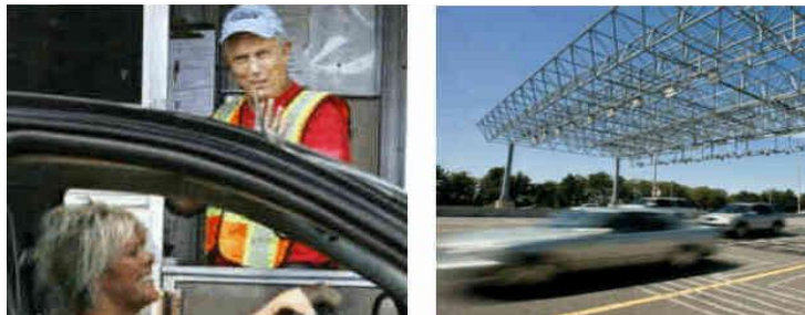
Traditional toll at left. Open road toll system at right, the Raritan Toll Plaza on New Jersey's Garden State Parkway. Sensors above read EZ Pass tags and license plates, collecting tolls at high speeds.
