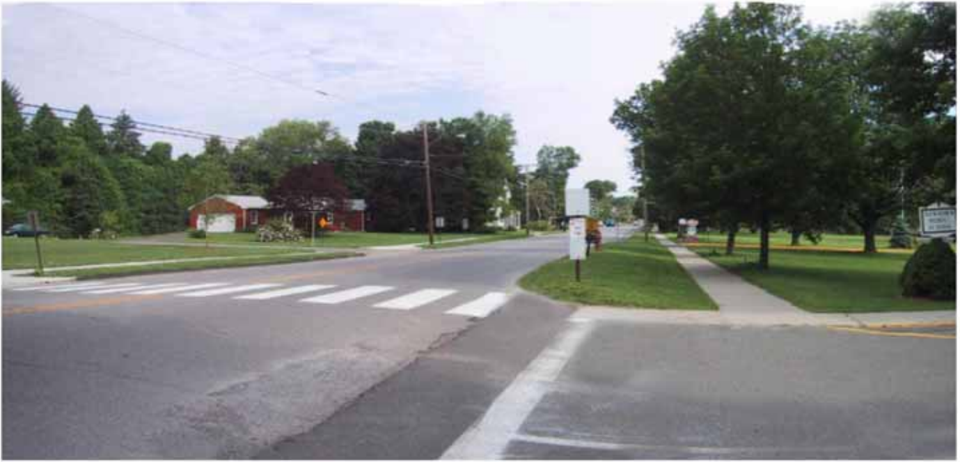
Existing: Queen Street mid-block crossing adjacent to the Middle School
