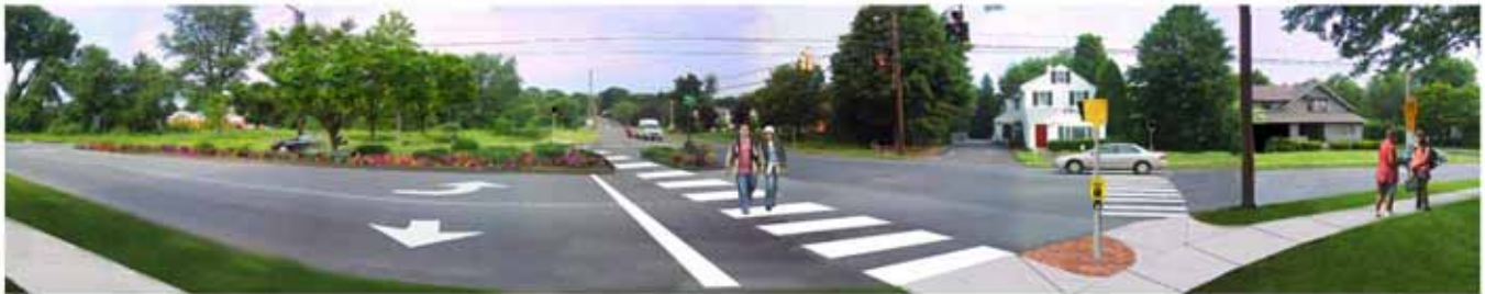
Proposed Enhancement: Gateway treatment, new crosswalk, pedestrian activation, improved sidewalk connections, and pedestrian signal indicators.
