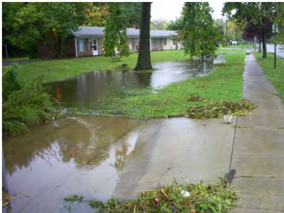
Photo 36: Overflow flooding downstream of culvert
