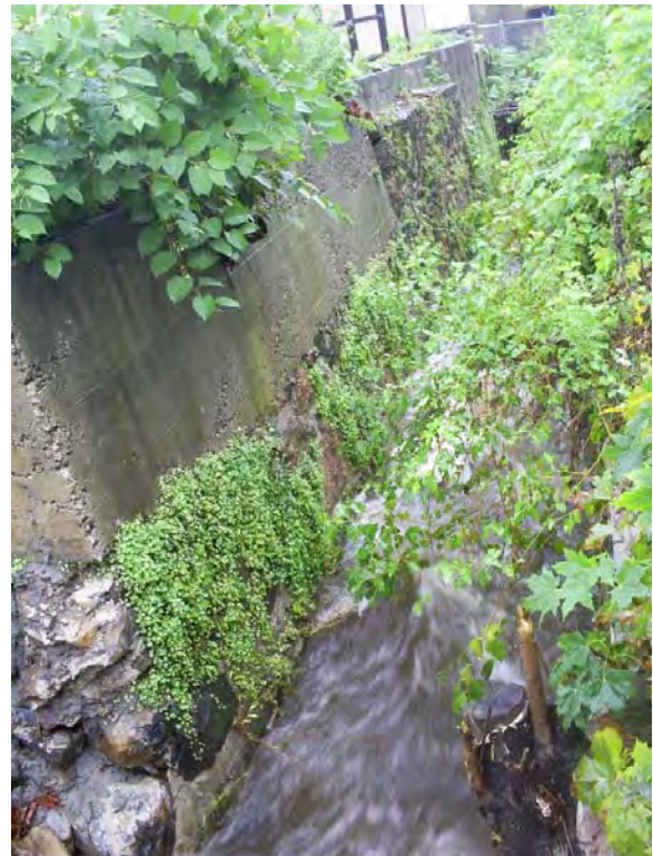
Photo 33: Blind Brook 2 nd constriction near shelter
