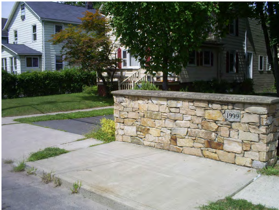
East Pearl Street bridge over Blind Brook culvert, replaced following Tropical Storm Floyd.
