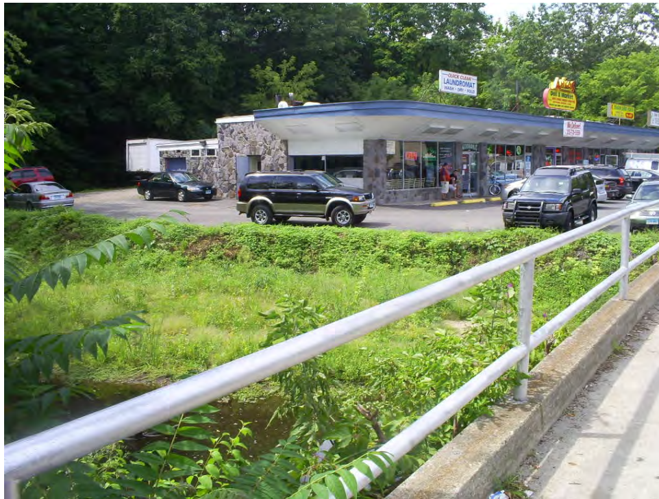
West Avenue bridge over Still River east of railroad tracks, looking west at Repetitive Loss Property.
