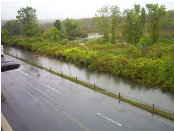
Photo 9: Mall drainage, berm, and Still River to NW
