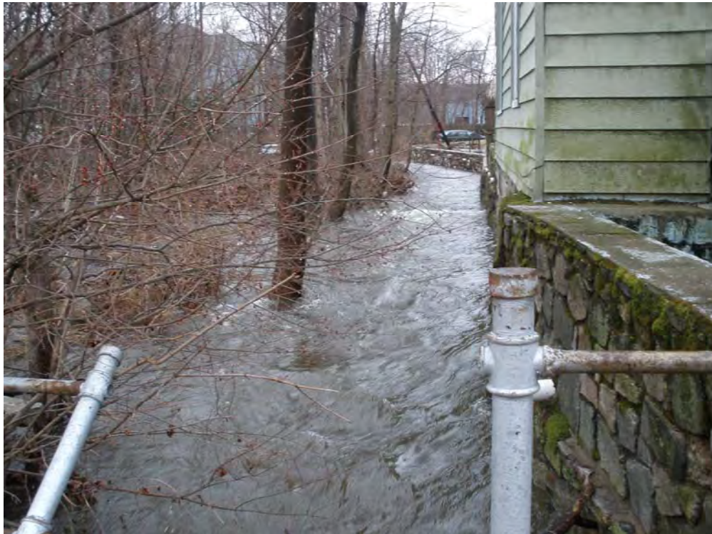
Blind Brook at George Street bridge, looking upstream
