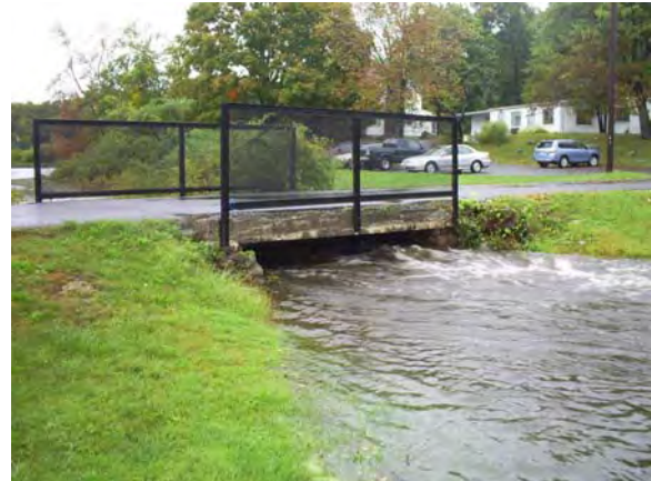
Photo 17: Downstream face of access road bridge
