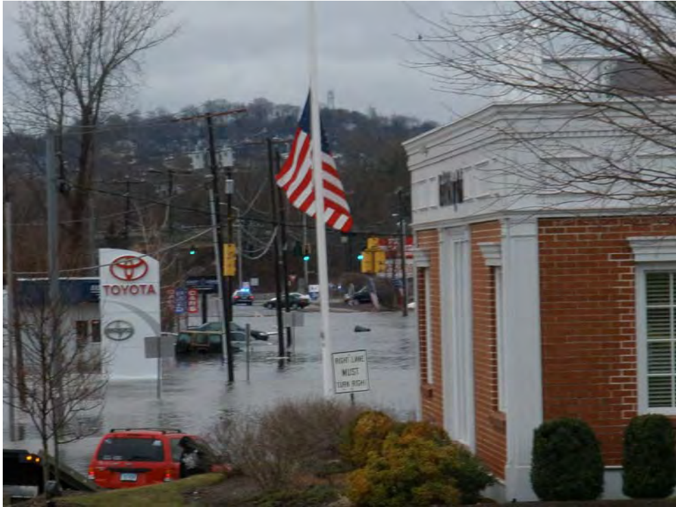
Still River overtopping Federal Road near Greentree Toyota. Note cars halfway inundated in background.
