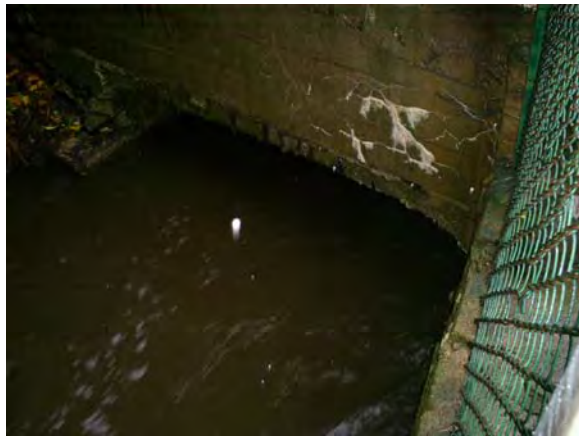
Photo 27: Blind Brook culvert daylight at Fire HQ
