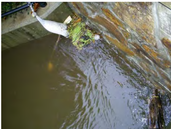
Photo 19: Upstream face of Blind Brook culvert
