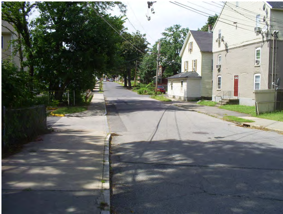
Repetitive Loss Property at 25-27 Patch Street (red door). Looking west from bridge over Padanaram Brook.
