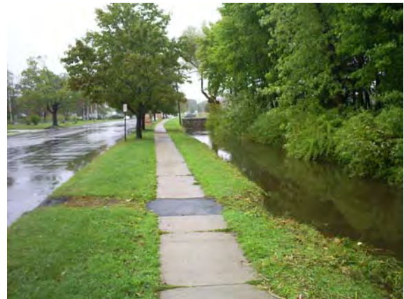
Photo 37: Memorial Drive swale looking upstream
