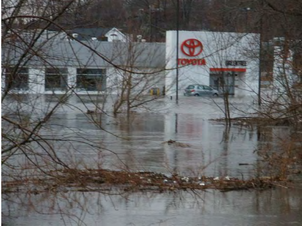
Still River flooding Greentree Toyota on Federal Road (Repetitive Loss Property)
