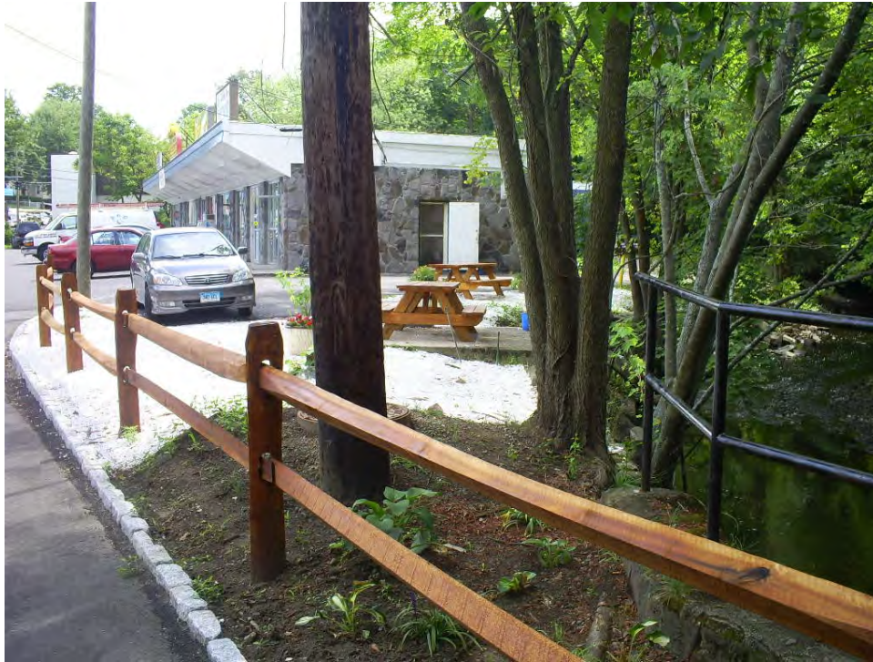
West Avenue beneath railroad overpass, looking downstream at Still River. Repetitive Loss Property is in background.
