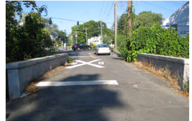
Depot Road Bridge Narrow bridge, lacks sidewalks and is insufficiently wide to carry traffic in both directions at the same time
