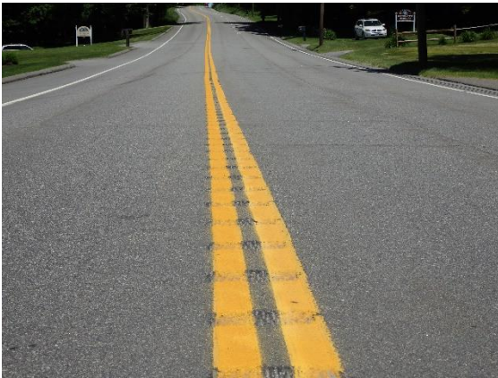
Figure 16. Centerline Rumble Strips (Source: CTDOT)
