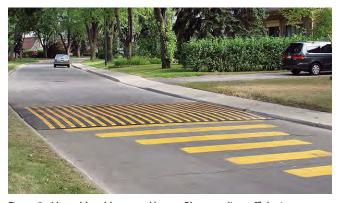
Figure 5 - Moveable rubber speed hump. Photo credit: trafficlogix.com
