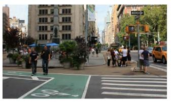
Figure 6 - Temporary bump-out in New York City consisting of paint and aggregate epoxied to existing street pavement. Photo credit: Dave Sousa
