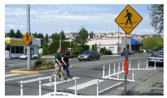
Figure 7 - Temporary Bump-outs consisting of paint, rubber curbs and flexible lane delineator posts. Photo credit: Road Safe Traffic Systems
