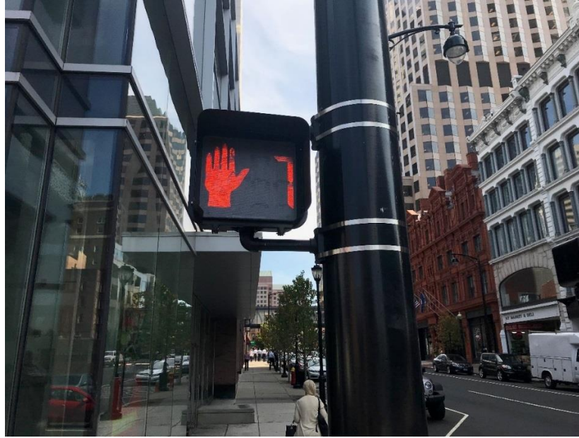
Figure 7: An APS signal with count-down timer in Hartford, CT (FHI)
