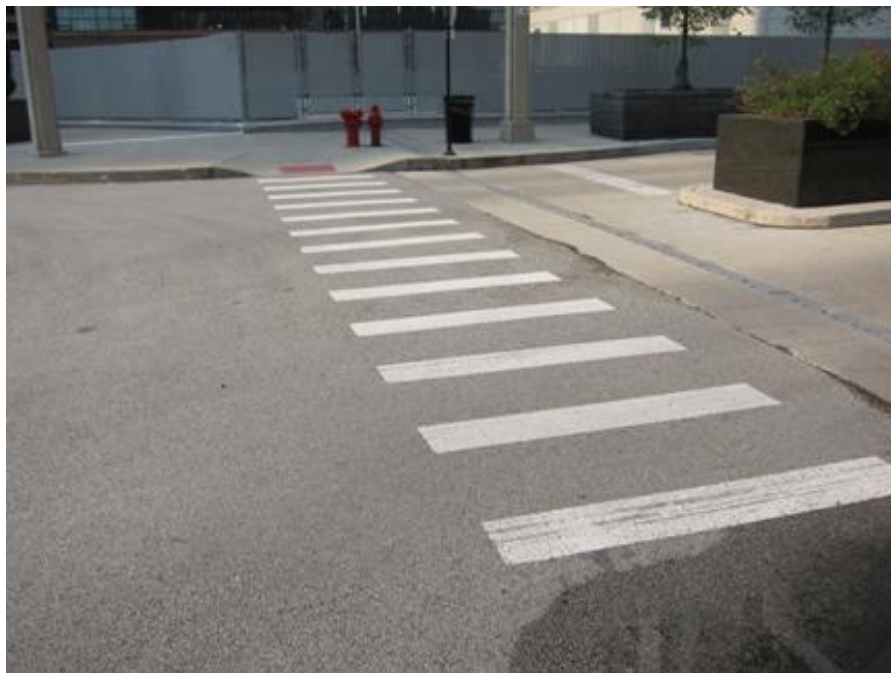
Figure 8: Continental crosswalks improve visibility of pedestrian crossing locations (FHWA)
