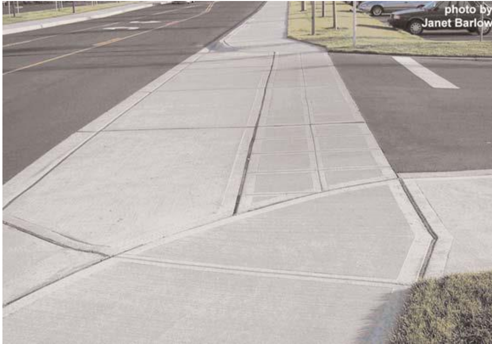
Figure 4: Concrete sidewalk continues through minor driveway (TRB, 2010)
