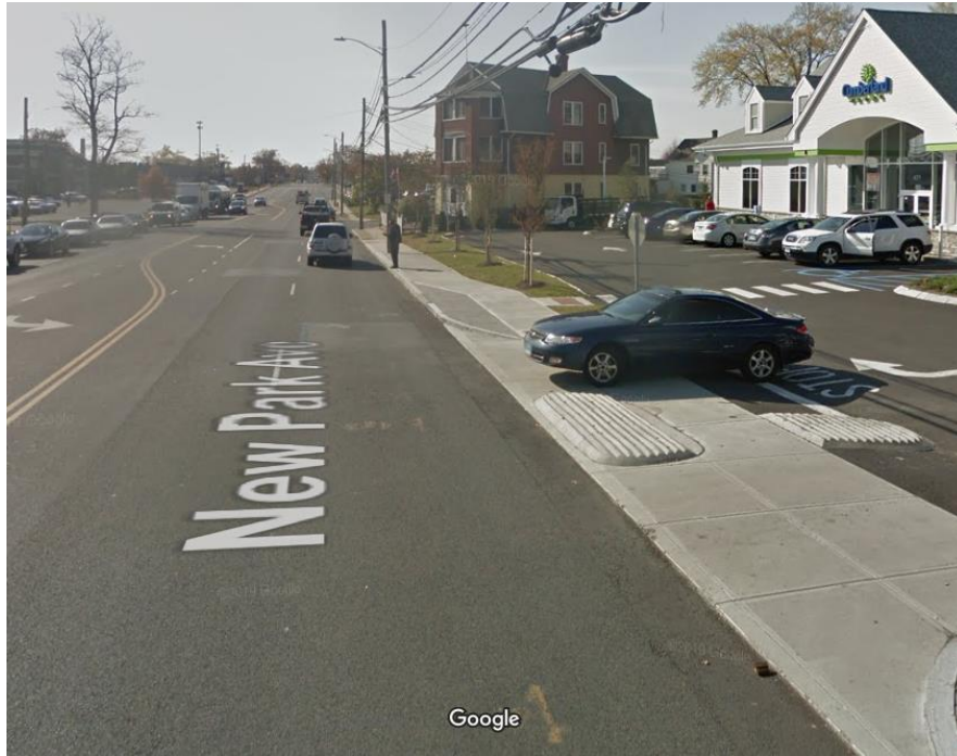
Figure 5: A truck-mountable channelized right-turn island located in West Hartford, CT on New Park Avenue (Google Maps)
