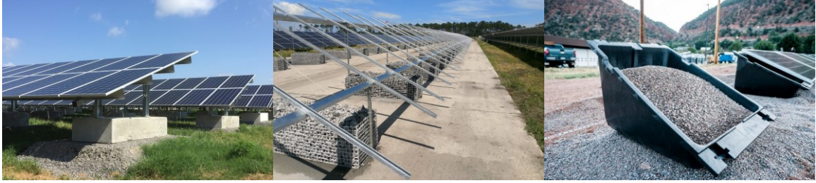
From left to right: Terrasmart (pre-cast concrete); APA ReadyRack Geoballast (gabions or rock baskets); Powerfield Energy PowerRack (polyethylene containers that can be filled with any ballast material)
