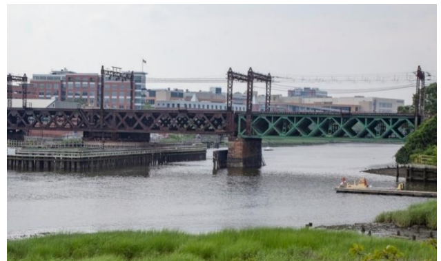
Walk Bridge Replacement
