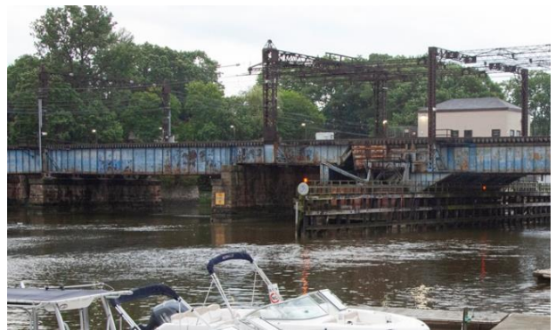
Saugatuck Bridge Interim Repairs
