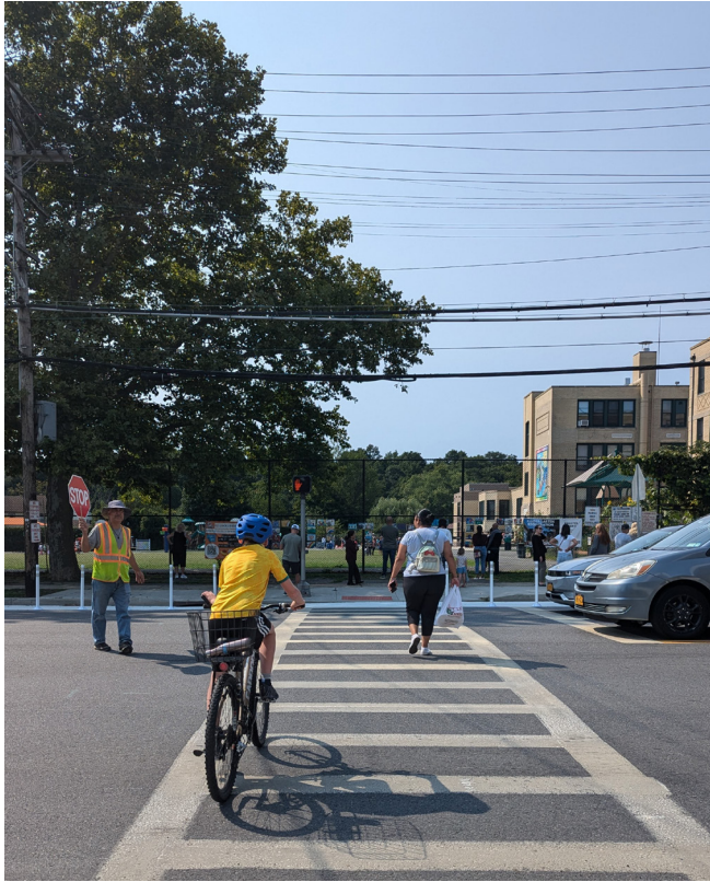
AKRF designed crosswalk curb extensions to improve safety for elementary school students crossing a wide arterial street leading to the Mamaroneck Avenue School.
