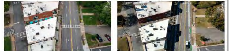
Before and after images of a lane reconfiguration project in Athens, GA
