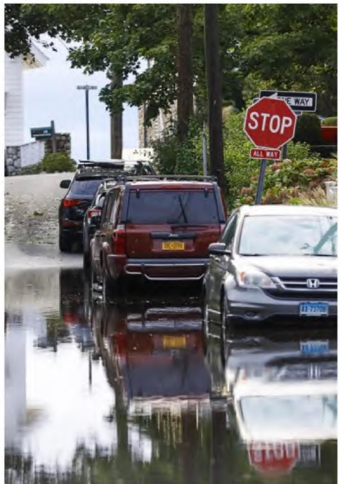
Flooding in Norwalk
