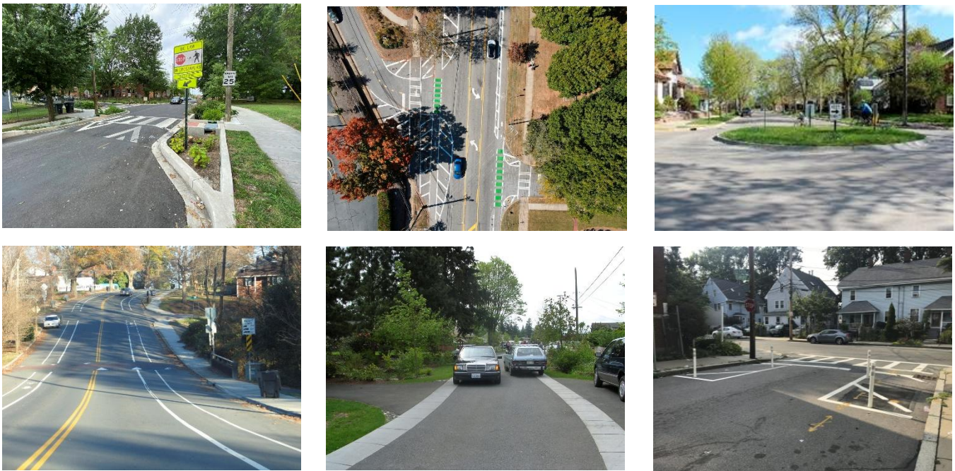
Figure 7 Raised crossing with stormwater infrastructure in Washington, D.C.; Intersection reconfiguration in Athens, GA; Roundabout in La Crosse, WI; Bike lanes and a speed table in Charlottesville, VA; Yield street in Seattle, WA; Daylighting treatments in Boston, MA
