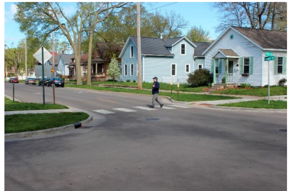
Figure 29 Curb Extension in a Residential Area of La Crosse, WI (Source: Toole Design)
