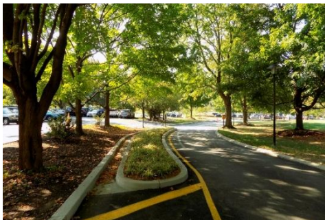
Figure 33 Example of a Lane Narrowing/Bump out treatment in Bethesda, MD (Source: Toole Design)
