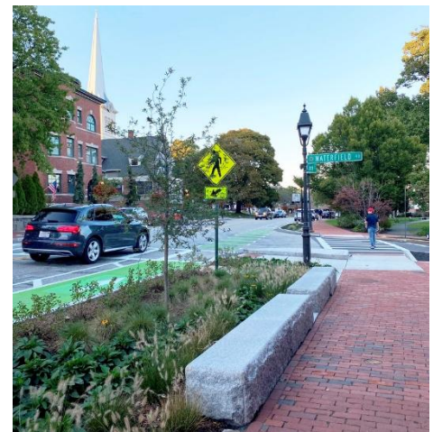
Figure 11 Stormwater Infrastructure in Winchester, VA (Source: Toole Design)
