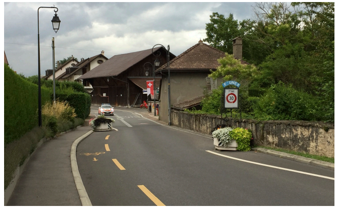
Chicanes in a transition zone in Founex, Switzerland
