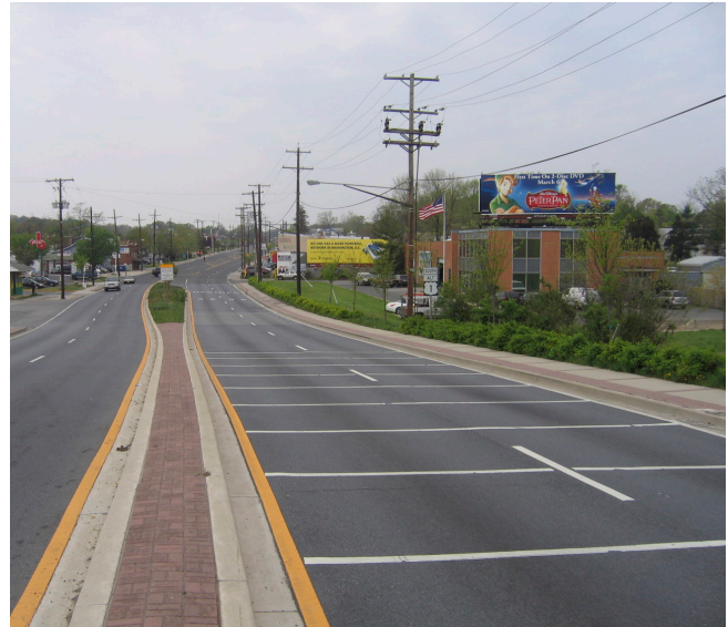
Transverse rumble strips and markings in Cottage City, MD
