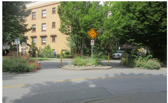
Diagonal diverter with landscaping in Vancouver, BC, Canada
