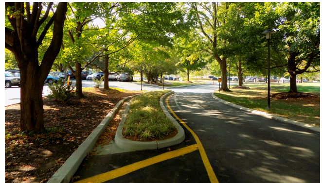
Lane narrowing paired with a physical bumpout in a School Zone in Bethesda, MD
