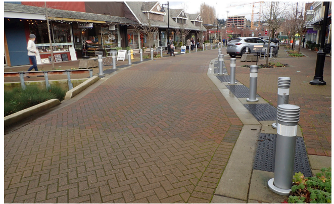
Bollards and parking provide physical separation in WA
