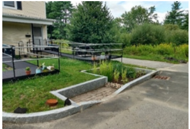
Green Stormwater Infrastructure
