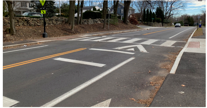
Speed table with a raised pedestrian crossing on Highland Avenue in Norwalk, CT (source: City of Norwalk)
