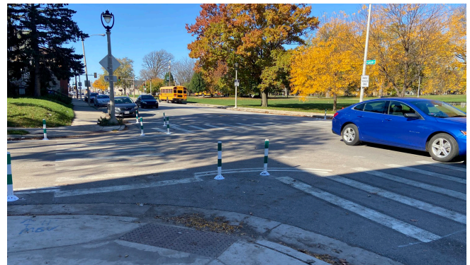
Low-speed curb radii with delineators in Milwaukee, WI
