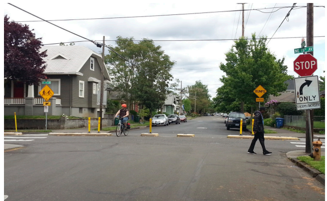
Median island with through-access for bicyclists on a bicycle boulevard in Portland, OR
