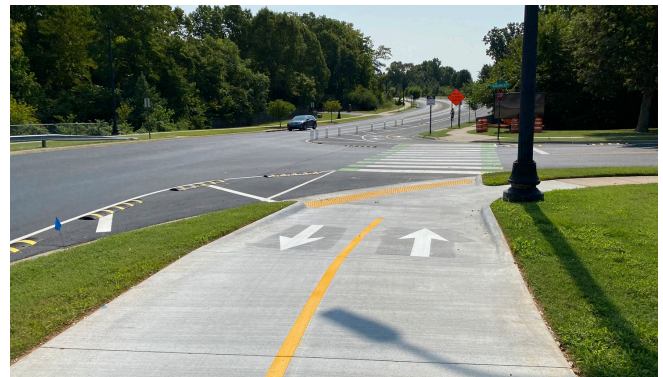
A quick-build example of low-speed curb radii in Bentonville, AR
