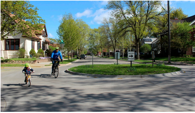
Mini-roundabout on a residential street (and bicycle boulevard) street in La Crosse, WI
