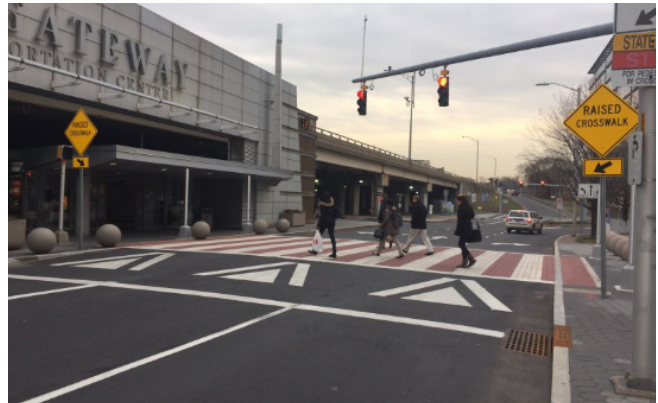
Raised crosswalk on North State Street in Stamford, CT (source: UCONN - CTI)
