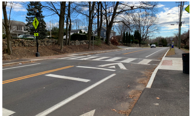
Raised crosswalk on Highland Avenue in Norwalk, CT (source: City of Norwalk)
