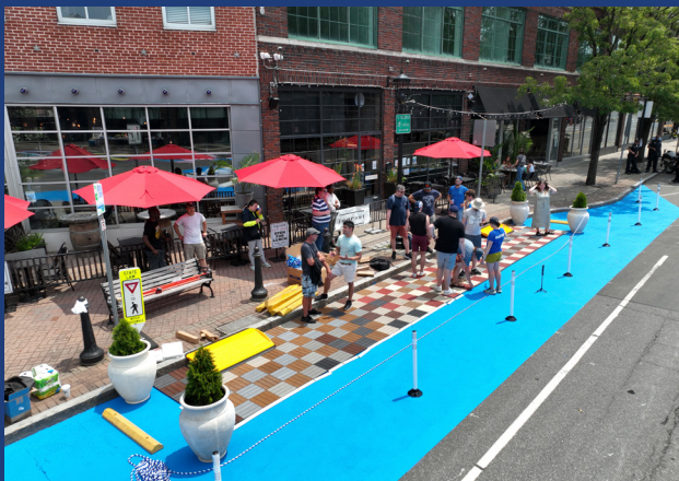
Example of a Demonstration Project in Norwalk, CT in 2024. Temporary traffic calming measures included painted curb extensions and a median island, as well as a parklet. (Source for both images: City of Norwalk)
