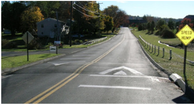
Speed hump on Larson Road in New Milford, CT (source: UCONN - CTI)
