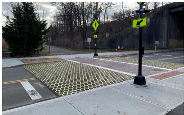
Raised crosswalk on Union Avenue in Norwalk, CT (source: City of Norwalk)
