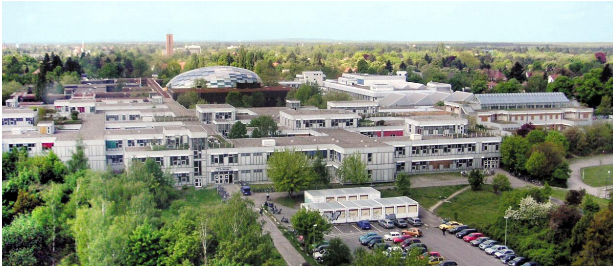
Figure 4. Example of modern, relocated structure (Freie Universität, Berlin)
