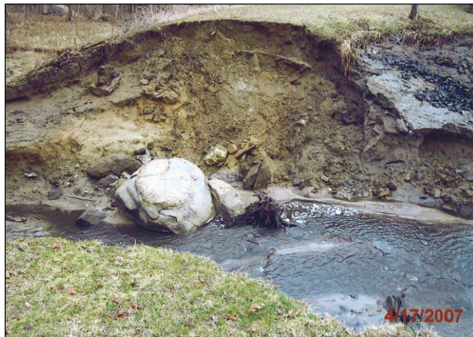
Figure 3-30: Rogers Pond Dam Breach in Sherman Source: Town of Sherman
