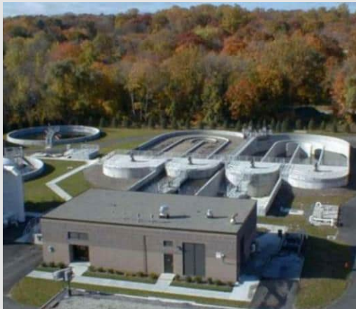
New Canaan WWTF
